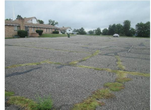
Parking spots can be replaced with porous asphalt to capture and infiltrate stormwater runoff from the parking lot. Two rain gardens adjacent to the building can capture, treat, and infiltrate roof runoff. A preliminary soil assessment suggests that more soil testing would be required before determining the soil's suitability for green infrastructure.
