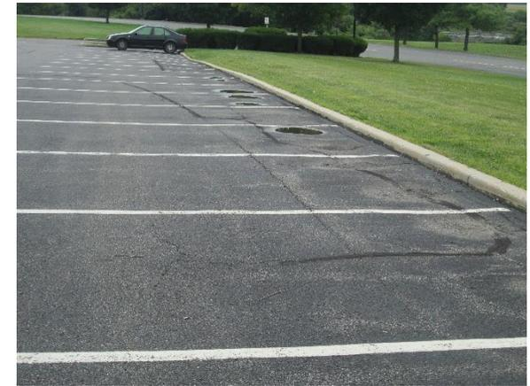
Parking spots to the west of the building can be replaced with porous asphalt to capture and infiltrate stormwater. A rain garden can be installed in front of the building to capture, treat, and infiltrate rooftop runoff. A preliminary soil assessment suggests that the soils have suitable drainage characteristics for green infrastructure.
