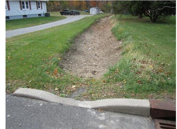
Rain gardens can be installed to capture, treat, and infiltrate runoff from the parking lot and roadway. A bioswale can be built in the ditch to the south of the basketball court to intercept runoff before it reaches the catch basins. A preliminary soil assessment suggests that more soil testing would be required before determining the soil's suitability for green infrastructure.
