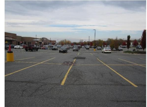
Bioretention systems can be installed along the northern end of the parking lot to capture, treat, and infiltrate stormwater runoff. Parking spots to the southeast of the building can be replaced with porous asphalt to capture and infiltrate stormwater. A preliminary soil assessment suggests that more soil testing would be required before determining the soil's suitability for green infrastructure.
